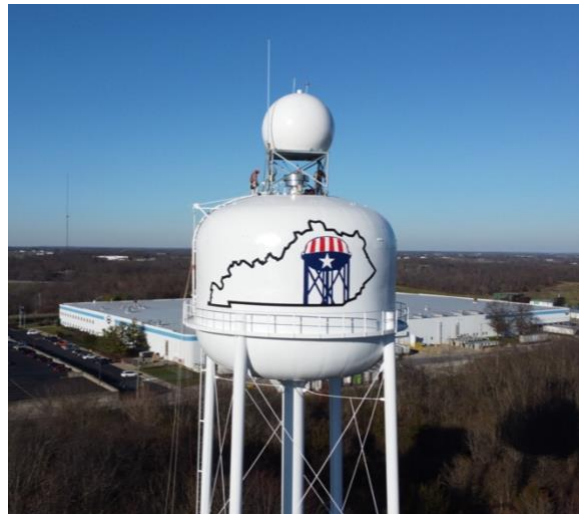
A Climavision X-band radar sits atop a water tower in Dry Ridge, KY
